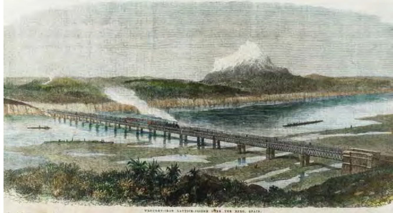
Wrought-iron lattice-bridge over the Ebro, Spain.
